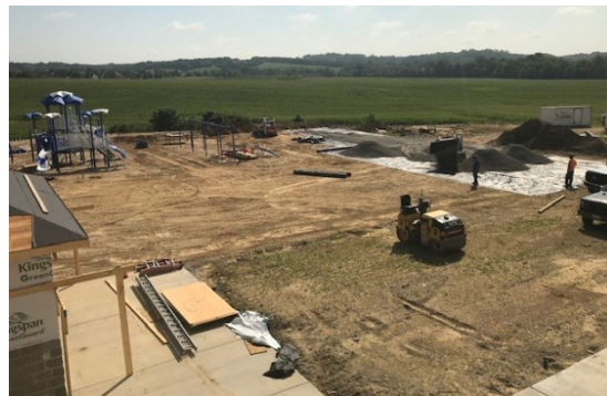
Rocking the base for the asphalt.
