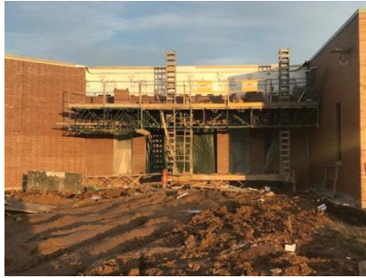
The last of the brick work!
